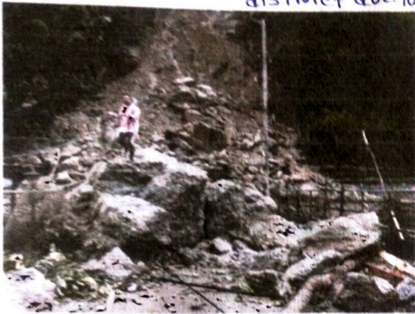
Teesta stage-v dam was broken due to landslides
